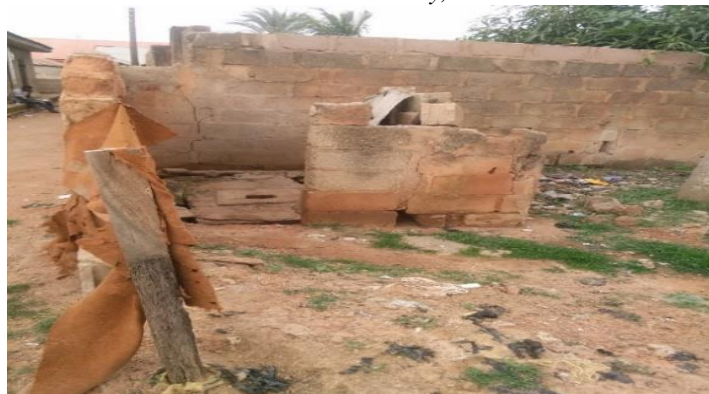
Plate 3: Collapsed Simple Unimproved Pit Latrine for in situ disposal at Sabo High Source: Field survey, 2020
